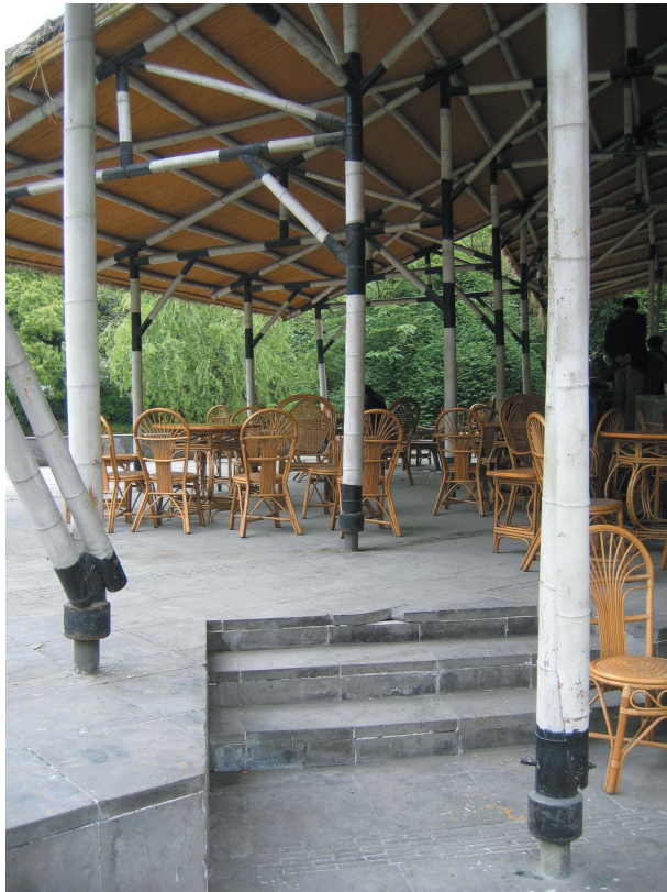
FIGURE 14. The usable space of Helou Pavilion (the painting does not completely match the original design proposal). (Photo by author, 2004).
